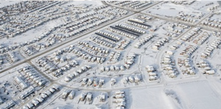
Drake Landing Solar Community, Alberta
